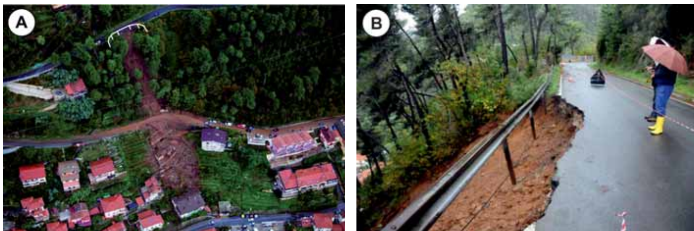
Figura 13 - A) Soil slip-debris flow triggered at Lavacchio, near Massa. It buried a house, killing two people. B) Detail of the crown.
