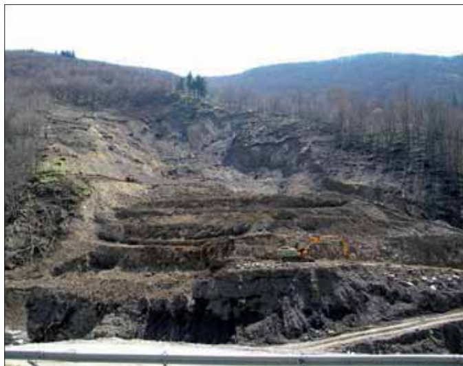
Figura 8 - Rotational slide involving fractured rock (sandstone and siltstone) and debris near Pracchia (Reno R. valley).
