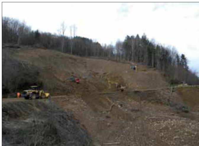
Figura 6 - Rotational debris slide triggered along the SR 445 road near Camporgiano village (Serchio R. valley).
